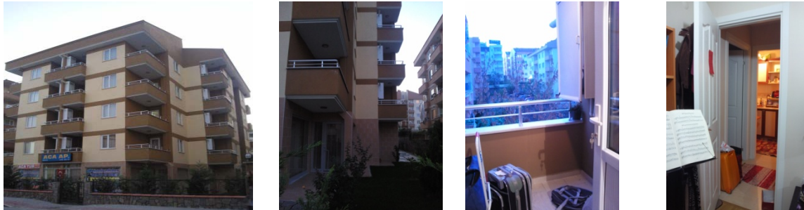
Image 2. Apartment A, view from inside and outside
