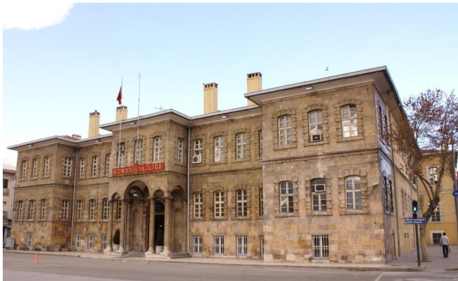
Figure 5. Today's photo of the building.
