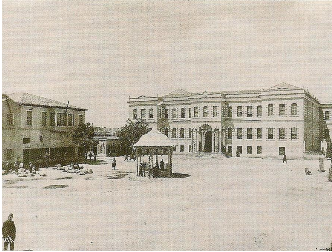
Figure 4. An old photograph of the building (Karpuz, 1998).
