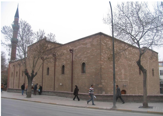
Figure 3. Today's photo of the building.
