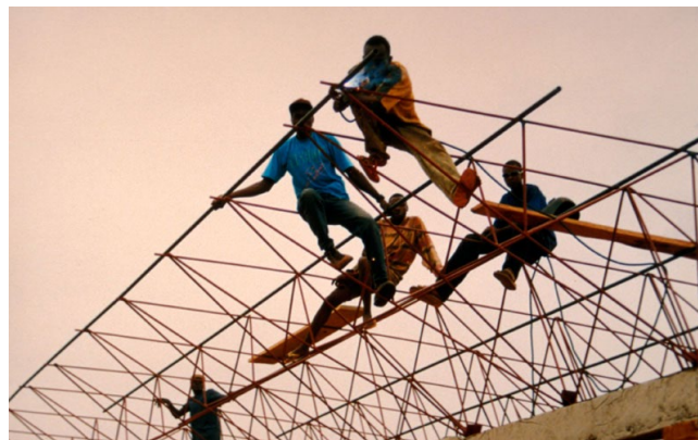
Figure 8. Workers assembling roof trusses, Photographer, Özgür Basak Alkan
