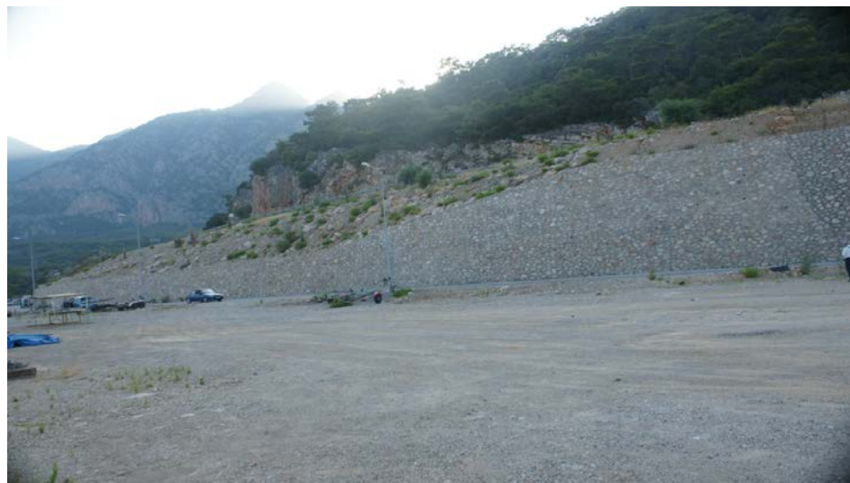
Figure 2. Left Side of Gravity Wall
